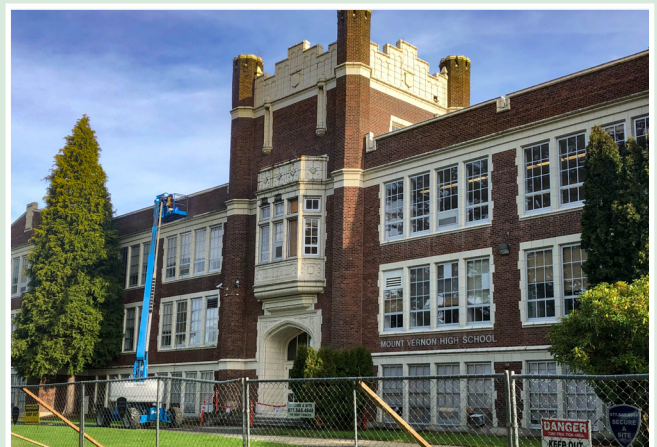
Construction site at Old Main on Mount Vernon High School campus.
